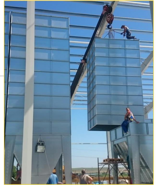
**Project:** 4 storage silos x 3900 tons + conveying equipment
