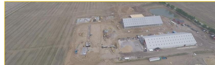
**Project:** 6 storage silos Frame x 3000 tons + conveying equipment up to 220 t/h, dryer up to 80 t/h
