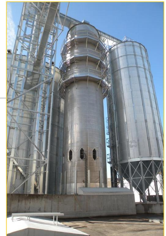
**Project:** 3 storage silos x 7800 tons + conveying equipment Skandia, tower dryer Sukup up to 150 t/h
