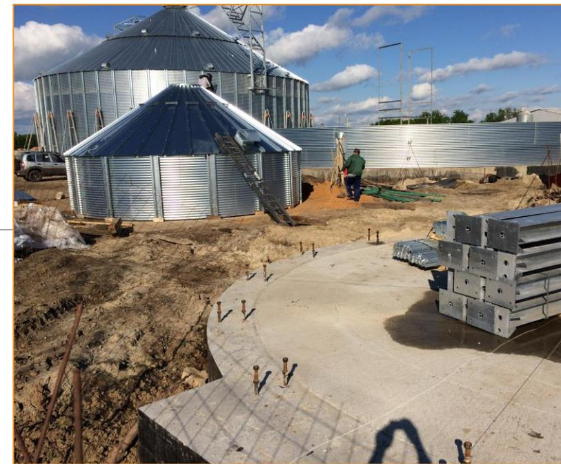
**Project:** storage silos 2 x 8000 tons, 2 x 5000 tons, 6 x hopper bins
