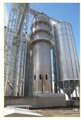
**Project:** 3 storage silos x 7800 tons + conveying equipment Skandia, tower dryer Sukup up to 150 t/h
